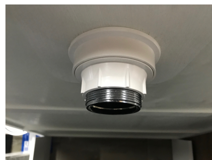
Shower waste assembled into the shower tray
