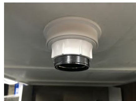
Shower waste assembled into the shower floor - rear view.
